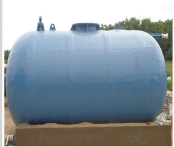
FRP Alum Storage Tank
