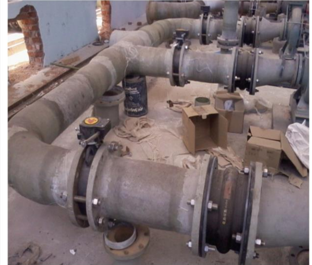
FRP Pipe Erections
